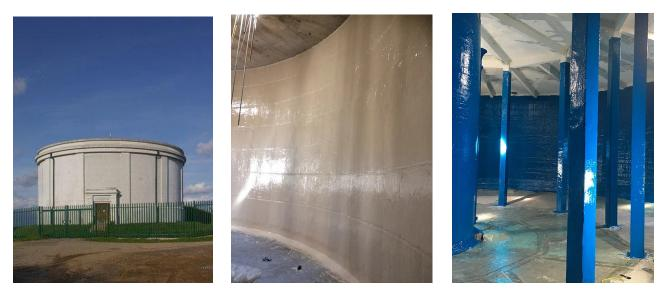
A full internal refurbishment was carried out to the walls, floor and shaft of the high level tank in this concrete water tower, in 2017.
