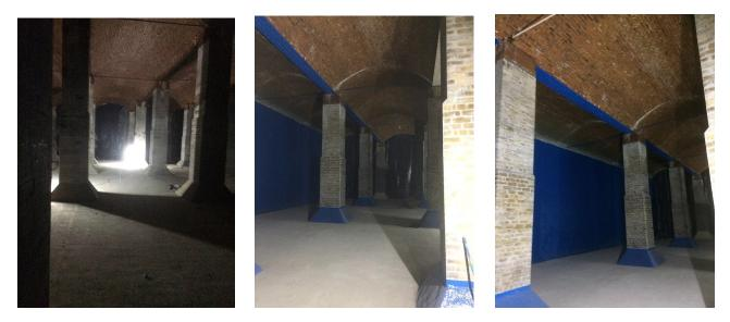
This enormous underground Victorian reservoir benefited from an extensive refurbishment in 2016, which along with the installation of a new external roof membrane, included the relining of the internal wall surfaces.
