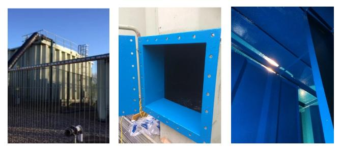
Acothane DW was chosen as the preferred water proofing solution for re-lining this above ground steel contact tank at a water treatment plant.
