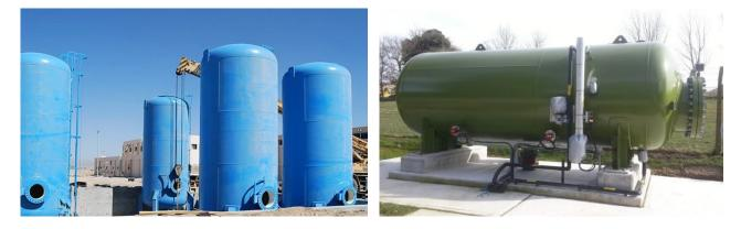
Surge vessels or pressure vessels play a very important role within the water industry with regards to assisting in the prevention of leakage from pressured water mains and preventing bursting pipe joints.
